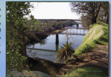
A view of the 700 foot long bridge from the Bluff.
