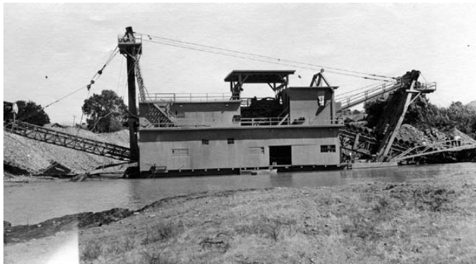
A dredger operating along the river
